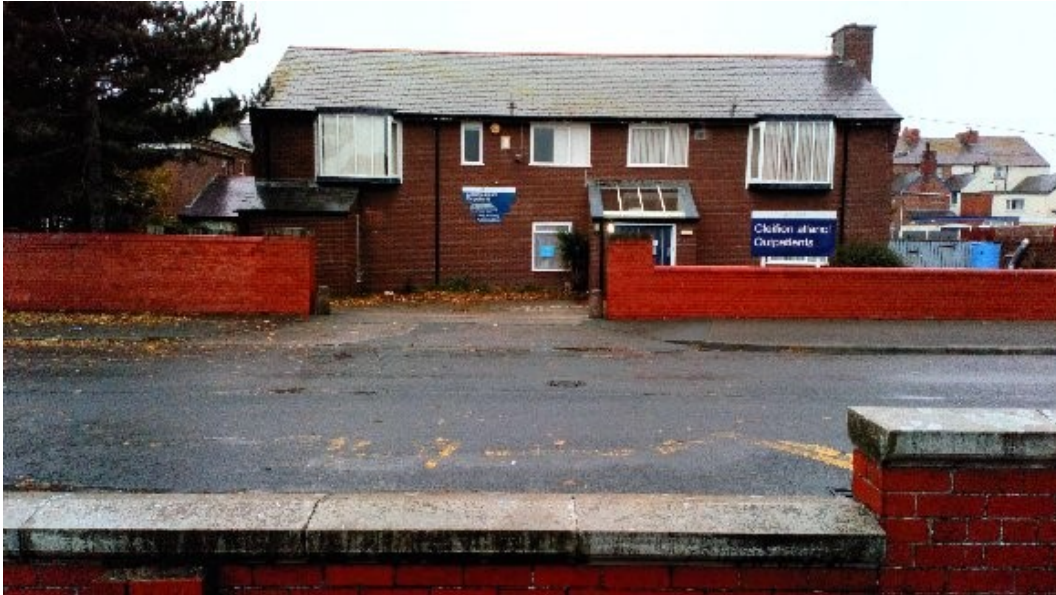
Figure 5: Photograph of Outpatient Department Temporary Building
